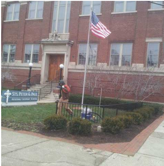
Above John's finished project of landscaping with flag pole, paving bricks and wrought iron fence.
