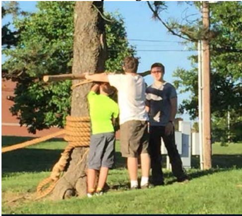
Above Ryan and Nate Carpenter and one other unidentified Scout building the monkey bridge.
